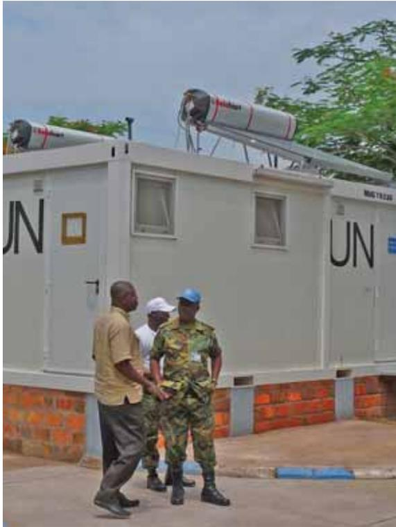
Solar water heaters are mounted on the roofs of sanitary units at a UN peacekeeping base in Kinshasa, DRC
