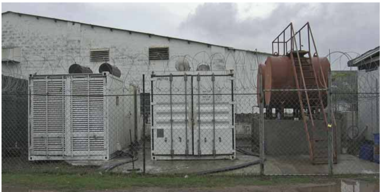
Proposed power is at the rate of 2 kW per person generated exclusively from a bank of diesel powered generators supported with 100% back up
