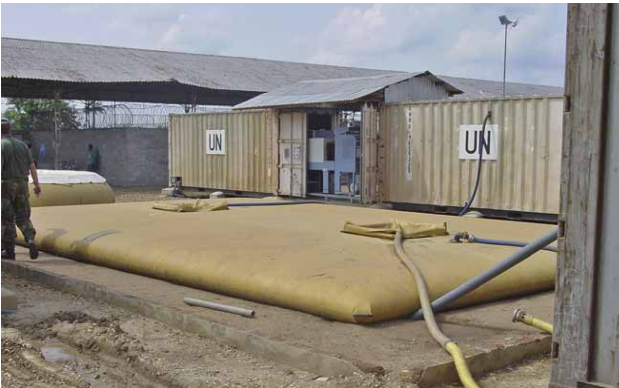
Water bladder installed by Troop Contributing Countries, MONUC, Kindu
