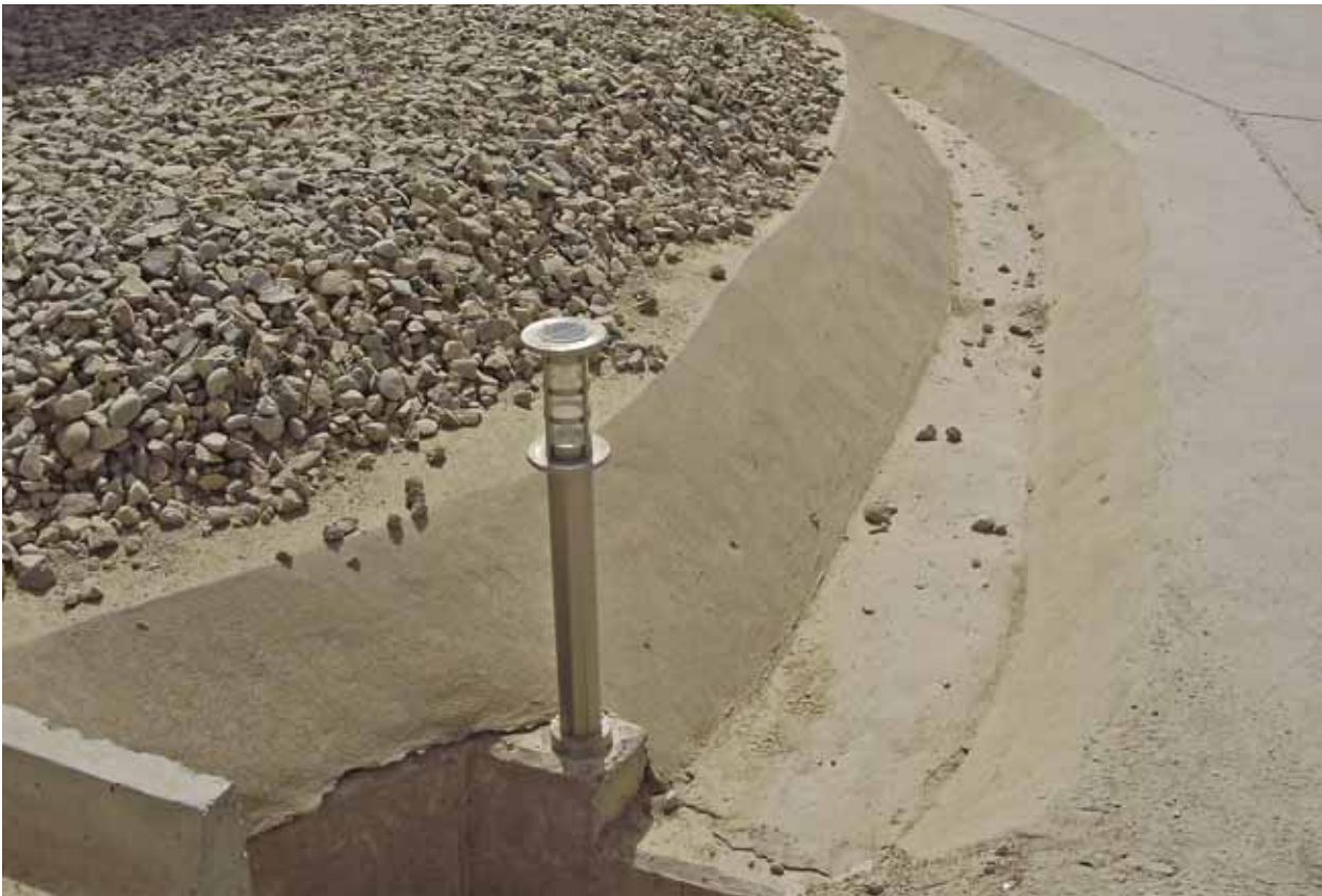
Stand alone renewable powered lamps (either photovoltaic or wind) offer security enhancement and potential cost savings due to decreased cabling costs and demand on generator fuel
