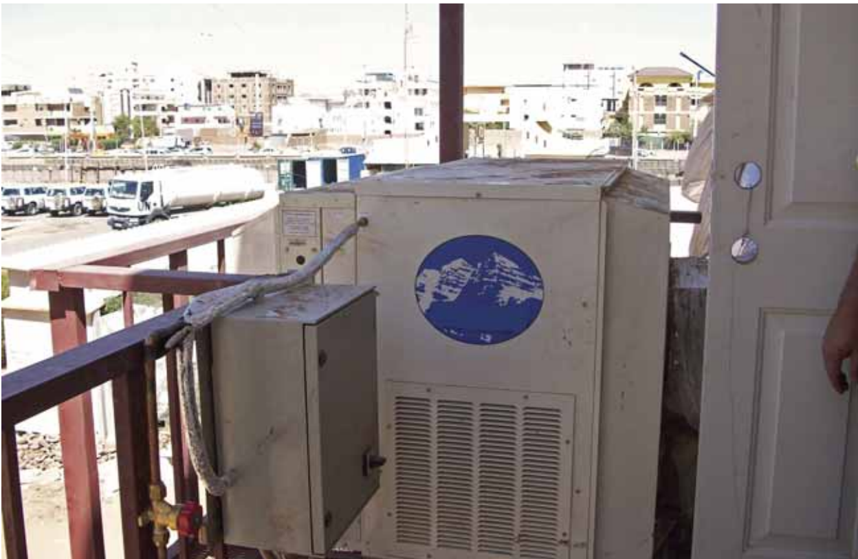
Coolerado-type, a new technology that makes use of the evaporative properties of water for cooling, is a very efficient technology in the right setting. It was assumed to be viable only for the Support Base in Mombasa, which has access to sufficient and suitable water resources
