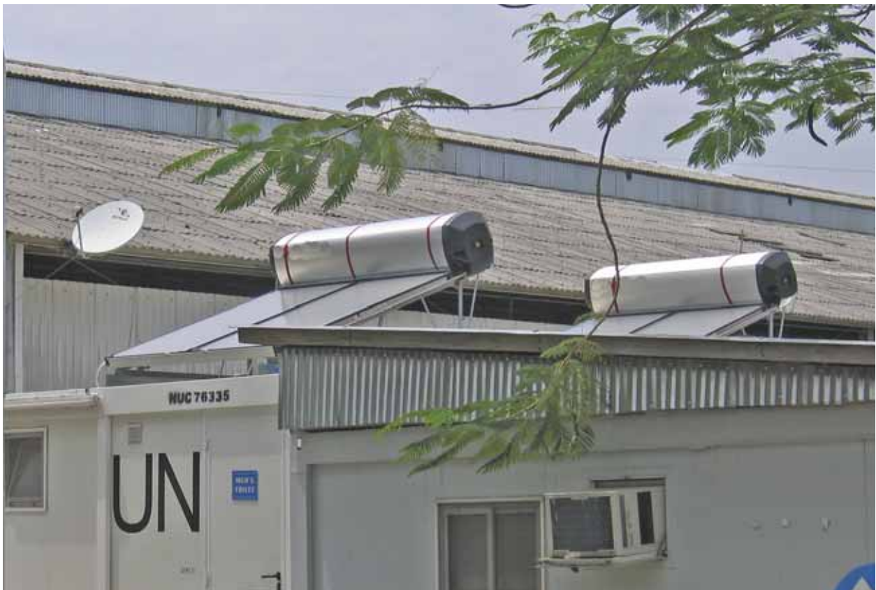
Solar thermal collectors, such as those seen on the roof of this ablution container in MONUC, Kinshasa, were ranked favourably as a low energy solution
