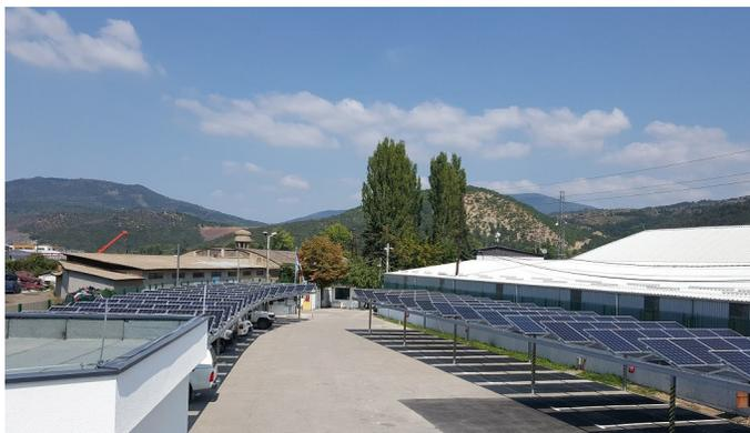
The UNMIK HQ in Pristina houses a fully functional solar PV system of 296 kWp integrated on the roof of the warehouse, with current production levels above expectations. Double glazed windows, light sensors in toilets and corridors, brightly painted interior walls, and centralized heating and cooling systems enhance the energy
